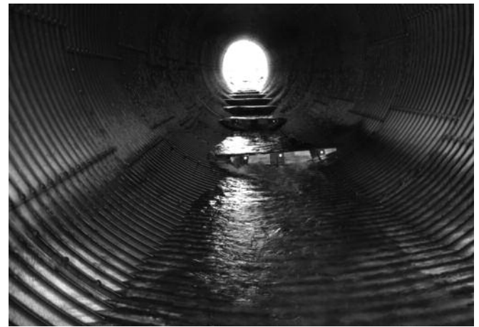
Looking upstream at the new baffles in the Mill Brook culvert.
