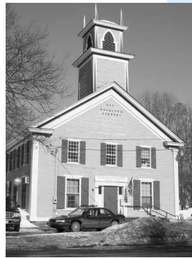
The new WRP office is on the second floor of the Royal Academy Building.
